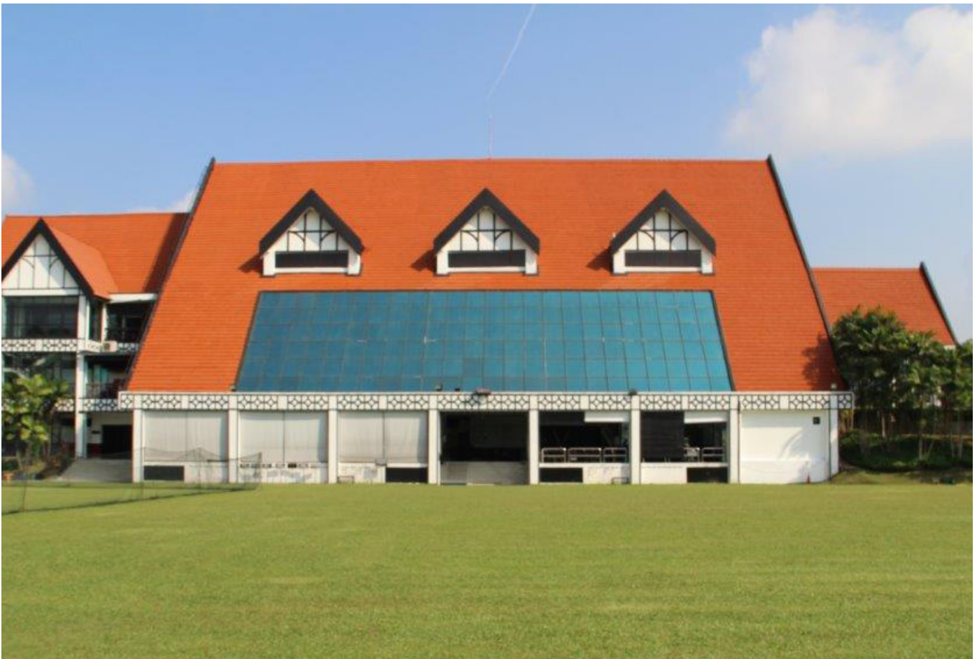
The spreuced up skylight slanting roof at Kiara
